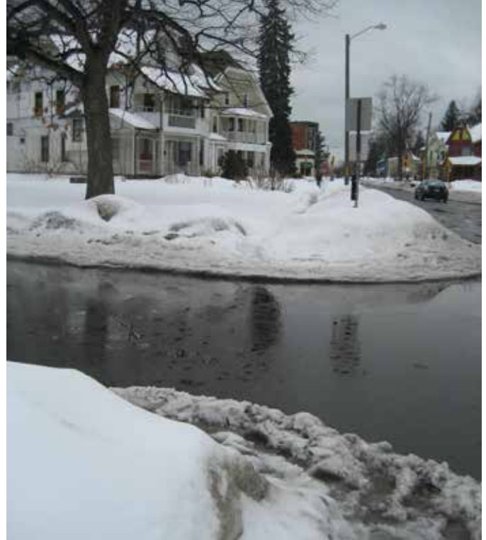
Bay Street was flooded where drainage structures were blocked by snow.
