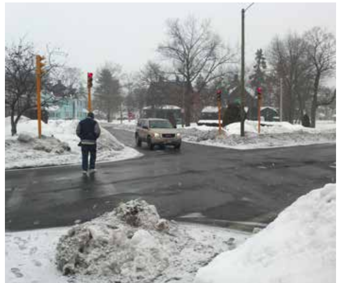
Catharine/Bay intersection has no pedestrian signals
