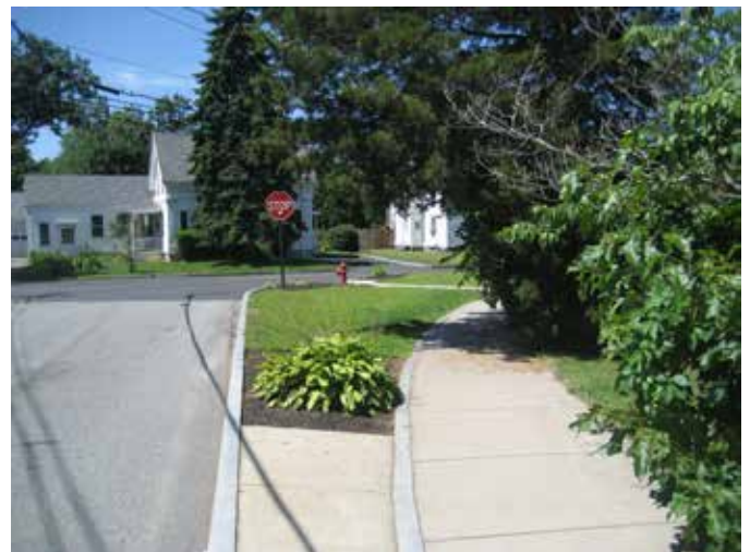
(B) Grass, trees and extended sidewalk in curb extension
