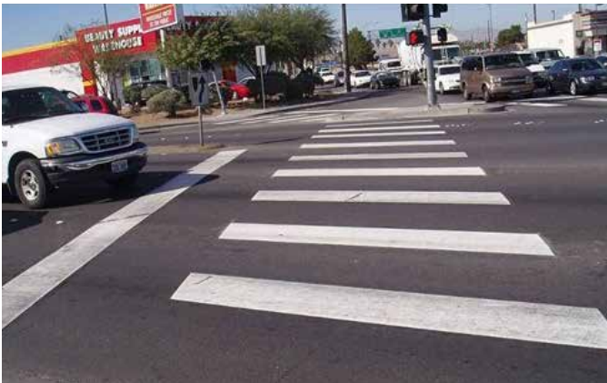
Crosswalk and stop line Source: http://safety.fhwa.dot.gov/ped_bike/tools_solve/ped_scdproj/sys_impact_rpt/images/fig16.jpg
