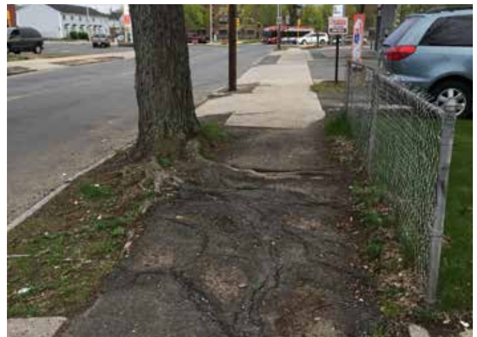
Tripping hazards like this one on Alden Street are common in Old Hill.
