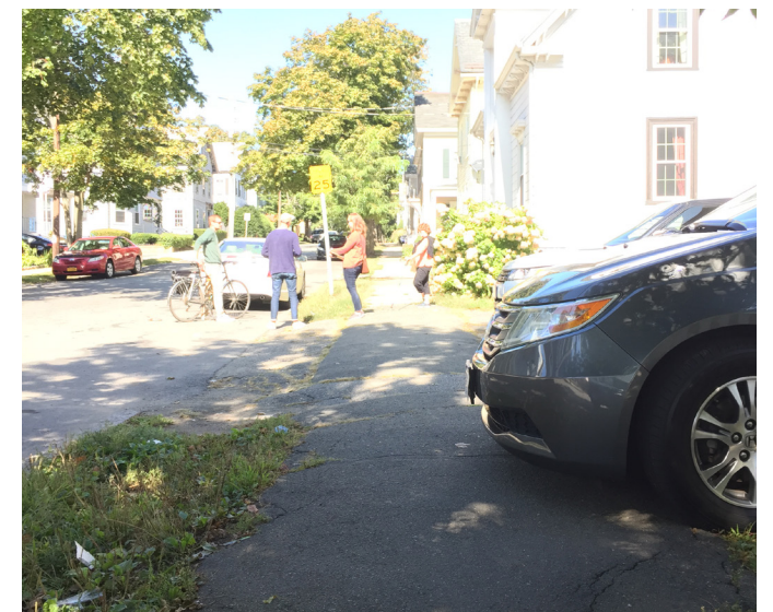
Poor walking conditions such as broken and cracked sidewalks, and obstructions like overgrown vegetation and cars parked into the sidewalk, are barriers for walkers along Buffum Street.
