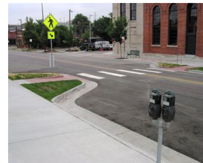
Curb extensions are often associated with mid-block crossings
