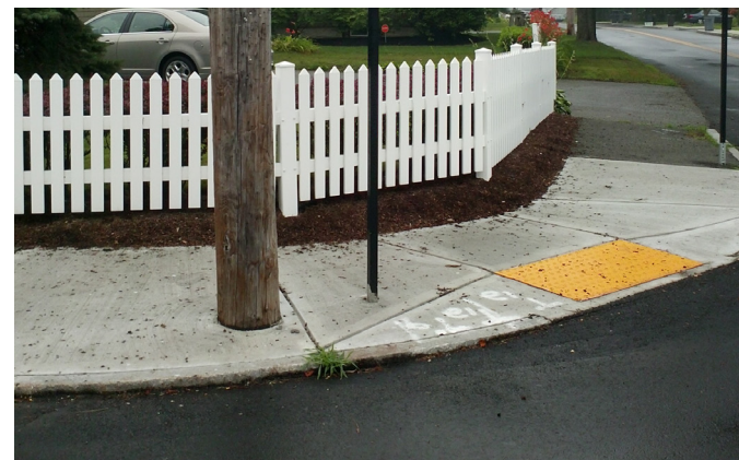
Curb ramp and detectable warning strip
