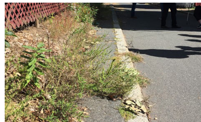
Overgrown vegetation on Randall Street is a challenge for walkers.
