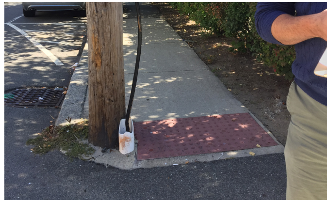
Power line poles on Mason Street obstruct the sidewalk.
